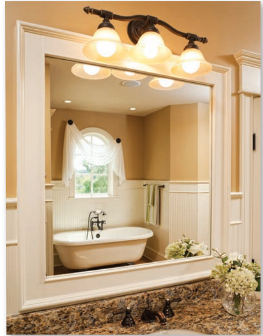
Wainscoting is attractive in traditional bathrooms and protects the walls from moisture.
